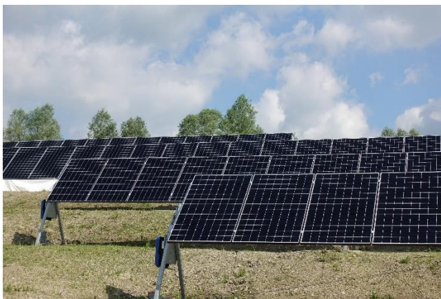
Photovoltaik-Anlage (Tracker)
